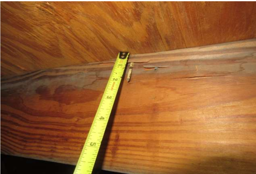
8d nails verified
